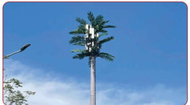
Trụ trang trí mỹ quan Camouflaged monopole tower
