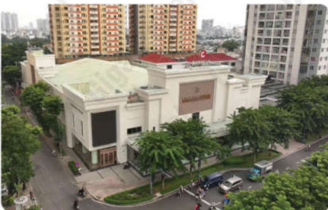
NHÀ HÀNG RIVERSIDE PALACE Riverside Palace Factory
